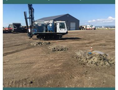
This drill rig ready to begin drilling a new hole. Piles of cuttings show the locations of recently drilled holes.
